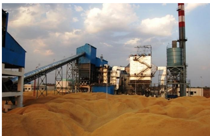
10 MW Biomass Power Project, Gadchiroli Distt. (Maharashtra State); Courtesy MNRE
