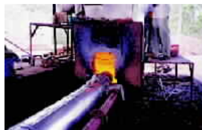
Gasifier with the heating furnace
