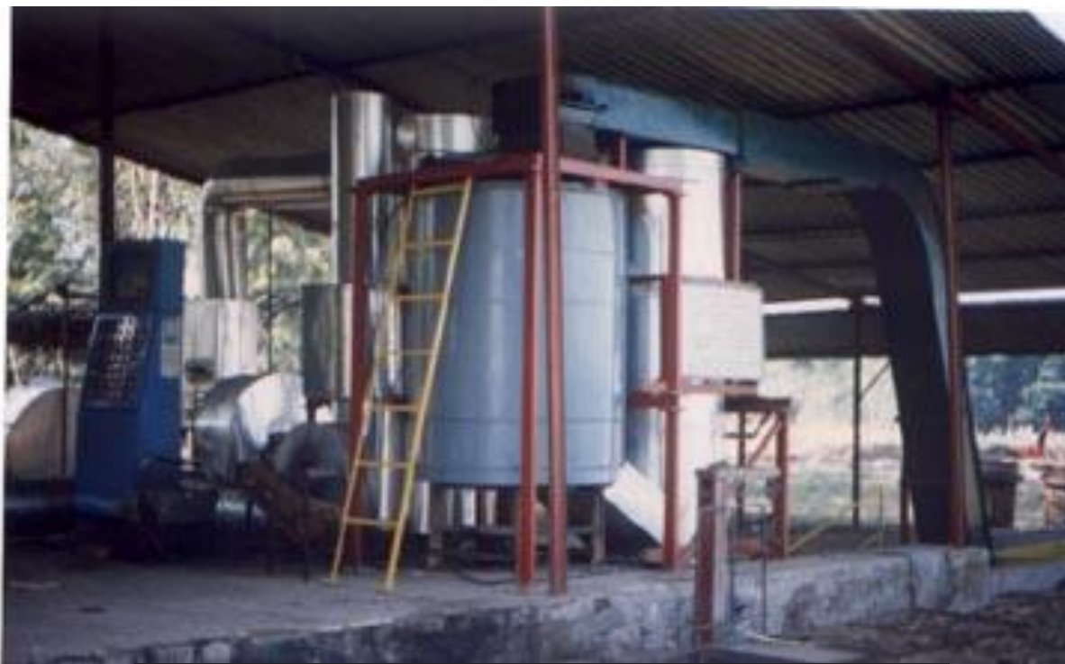
500 kW(thermal) loose biomass gasifier at NARI, 1997
